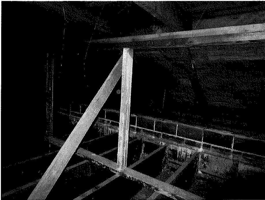
Figure 4: Typical Classroom Framing
