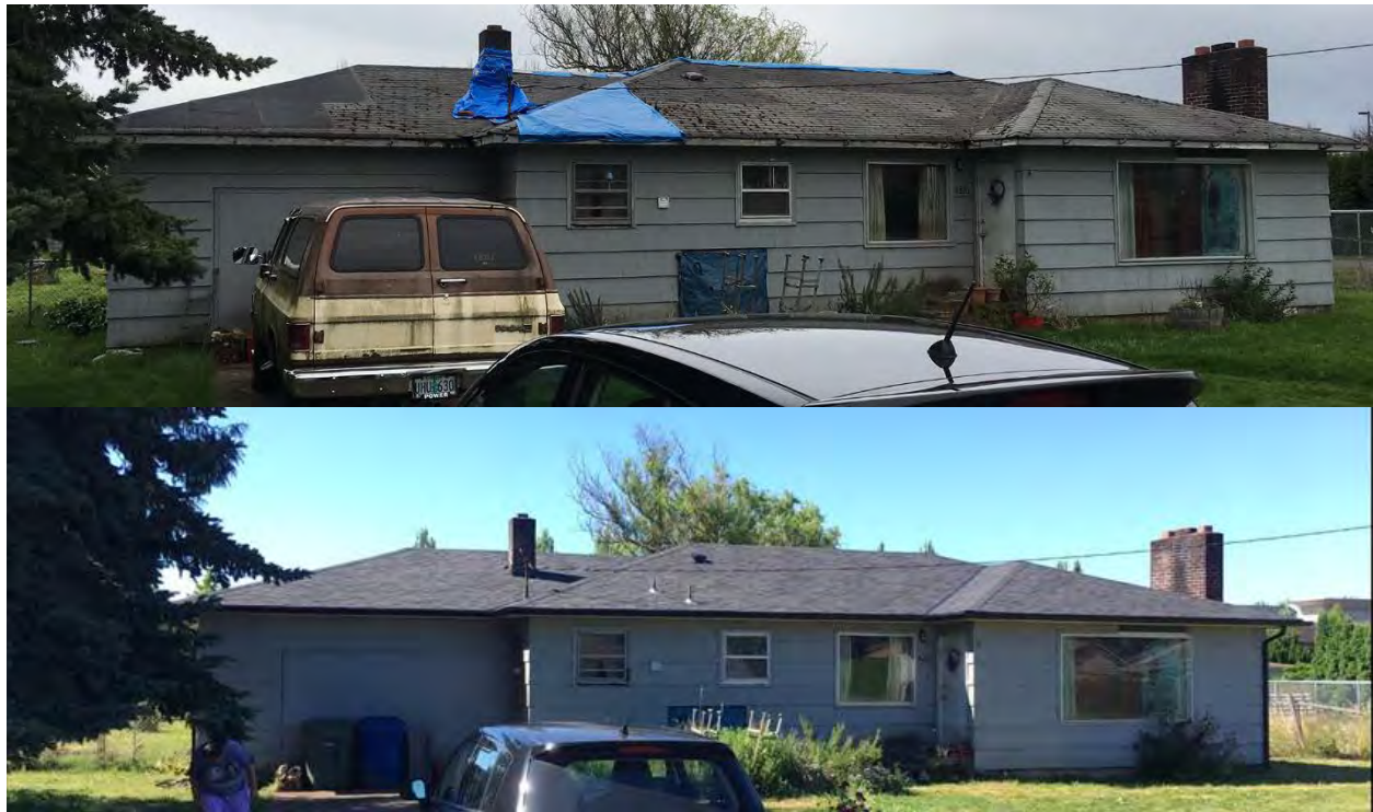
Above: Before and After where a homeowner in unincorporated Marion County received a new roof and repairs to interior drywall resulting from previous leaks from the damaged roof.
