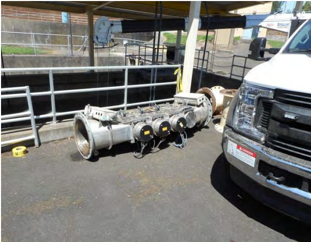
The old reactor chamber has been removed from channel 1.
