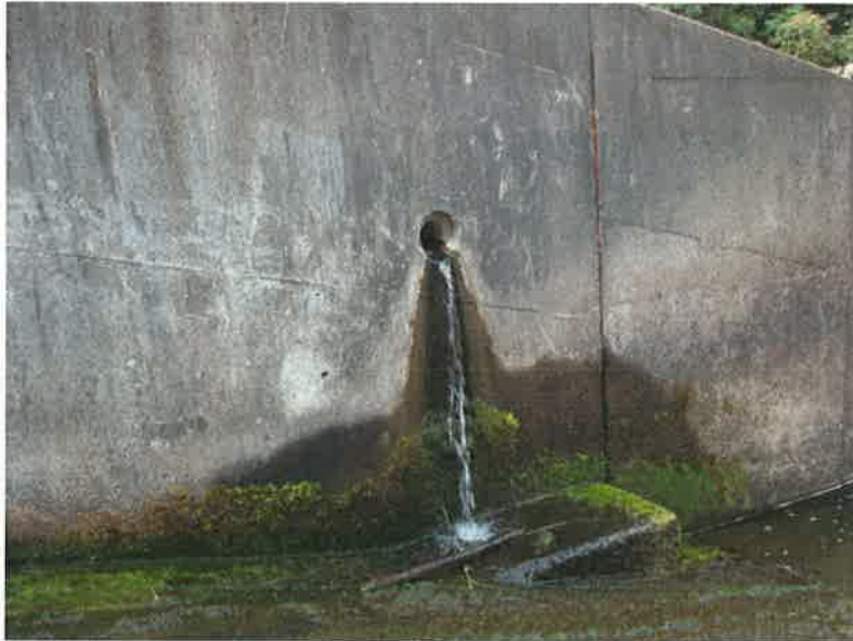
Spillway drain
