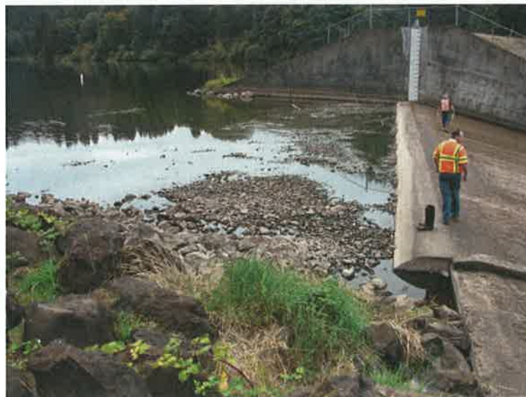
Spillway control section
