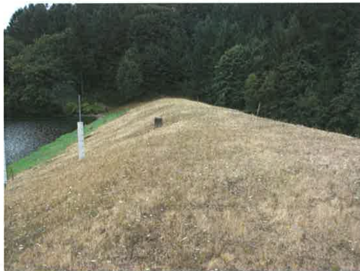
Crest and upstream face
