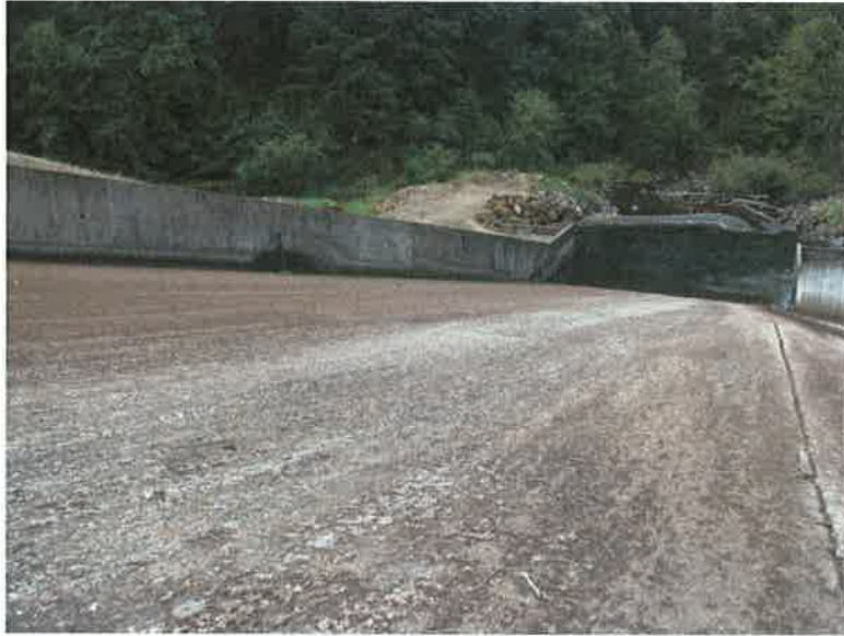
Spillway discharge channel
