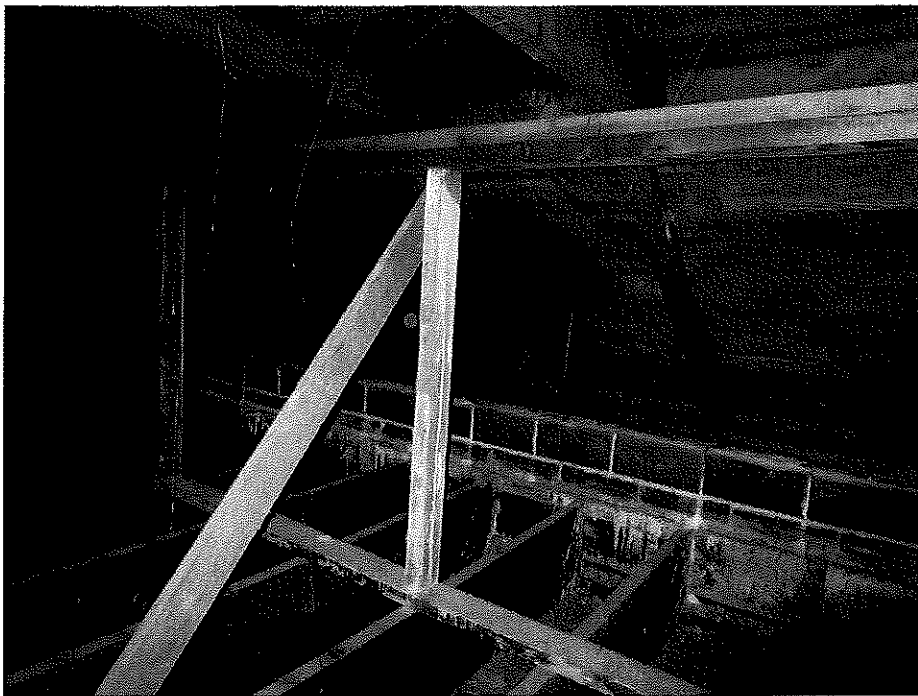
Figure 4: Typical Classroom Framing
