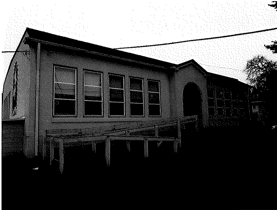
Figure 7: Classroom Wing Addition
