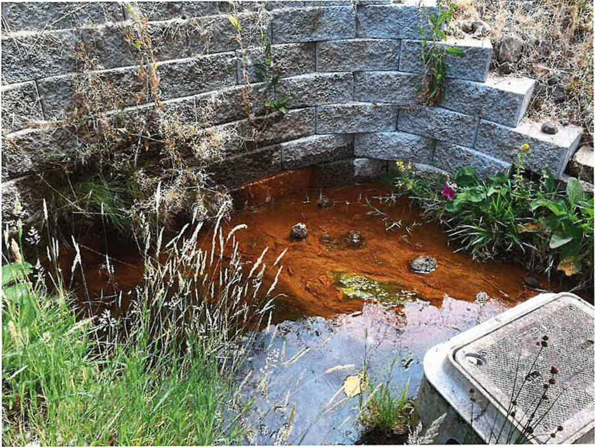
Typical seepage observed at reinforced area
